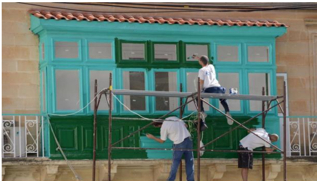
Three men at work restoring and painting a traditional wooden balcony in Sliema . Photo: Matthew Mirabelli
