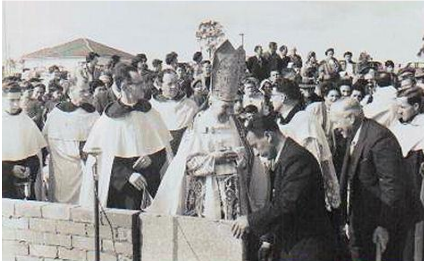
1Frank Cefai, Master builder, laying the foundation Stone of the Greystanes Church
