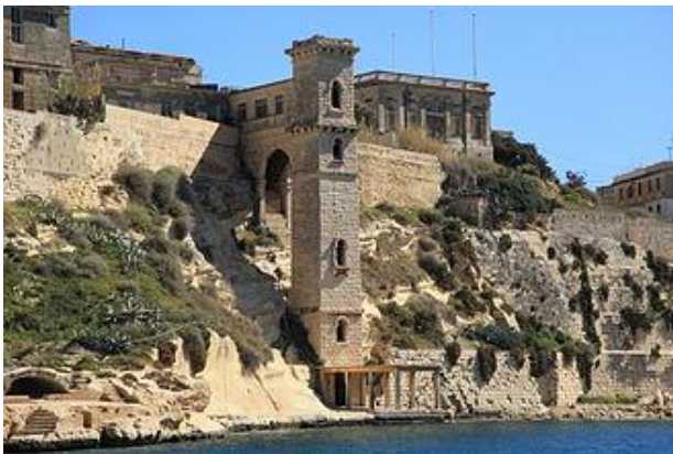
The Cot Lift at Bighi hospital in the middle.
