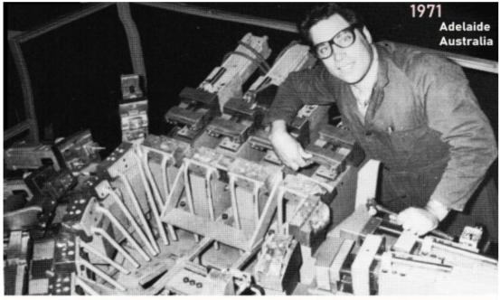
VINCE ZAMMIT (27) Toolmaker at General Motor Holden, ADELAIDE, working on a complicated die which is part of a unit to punch holes in the interior of car doors. Mrs Zammit (22) works at Gerrad Industries.
