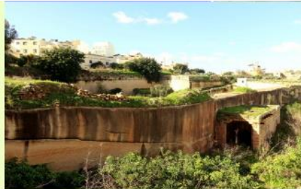
This quarry wall will be demolished and the site developed. Photo: Din L'Art Helwa.
