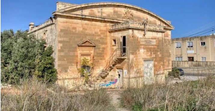
THE REMAINING CARCASS OF THE ICONIC ANZAC BUILDING IN MALTA
